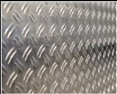
Floor plate covered with aluminium chequer plate
